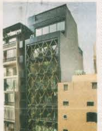
CHEHADE STREET A residential building built in 2008. The east-facing facade was fully glazed to get the maximum light in an otherwise densely built-up neighborhood.
