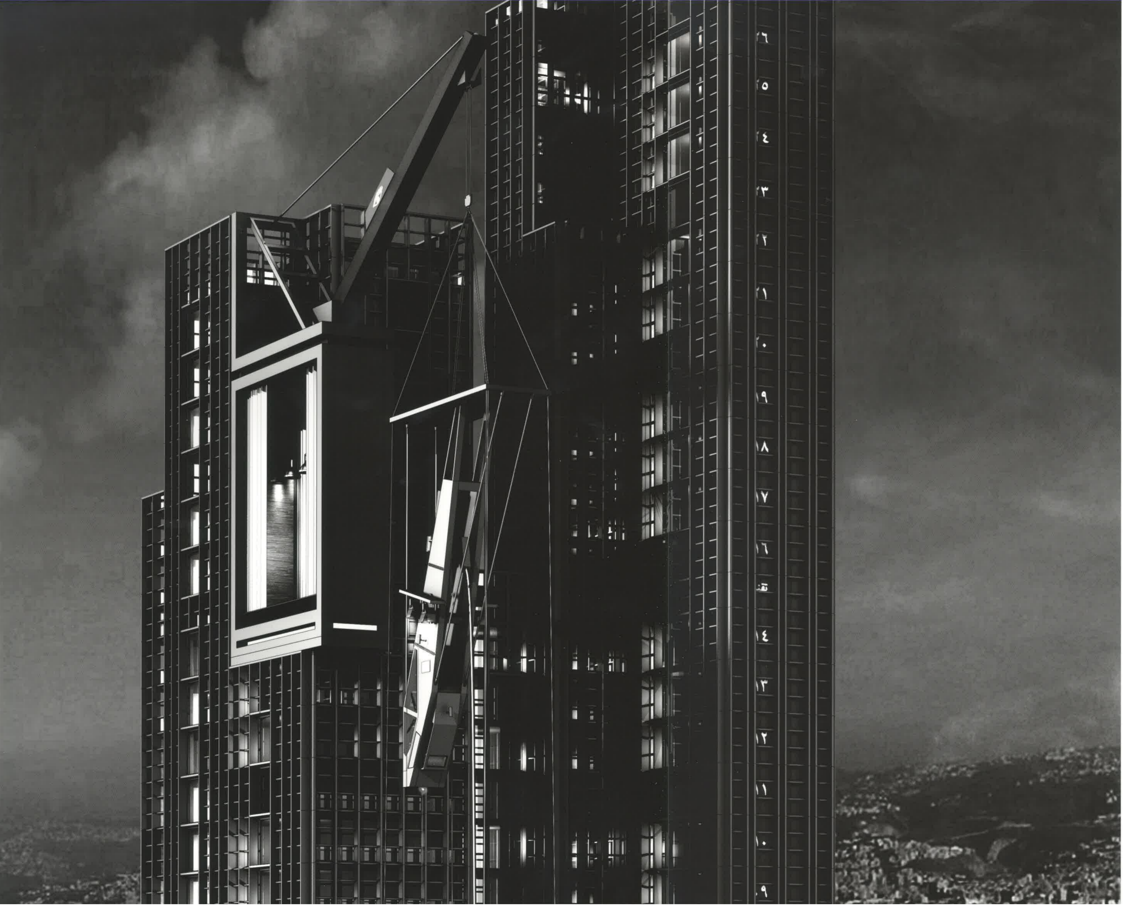
Plot # 450, which will be completed this year, Beirut 2019 ©DW5 Bernard Khoury
